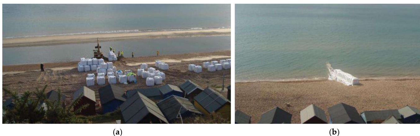
Figure 3. Pictures from the top of Hordle Cliff of (a) groin construction, filling the geobags during low tide on 27 September 2007; (b) view of the temporary structure deployed at Milford-On-Sea.
