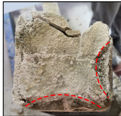
Fig. 9 arching effect in the cross-section of the column
