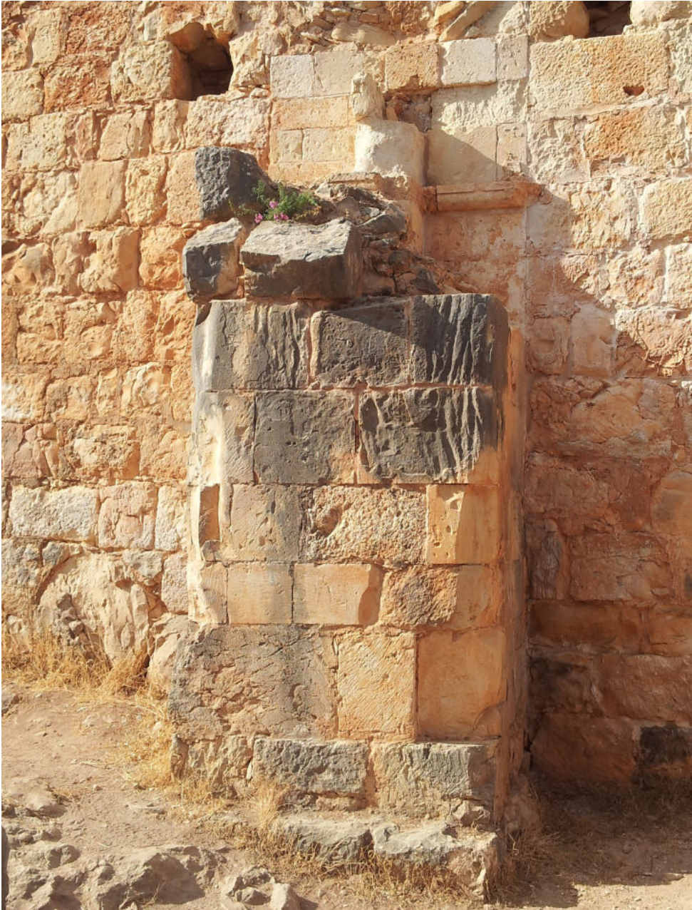
Fig. 16: Strengthening of the domestic ward structure (© Adrian Boas and Rabei Khamisy).
