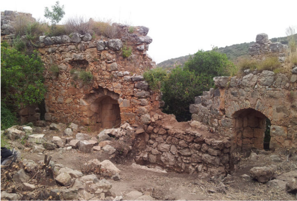
Fig. 3: Temporary wall blocking the space between the old outer wall and the new one (© Adrian Boas and Rabei Khamisy).
