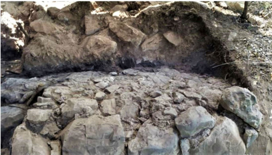
Fig. 20: Undermining of the domestic building (a) and the westernmost building (b) (© Adrian Boas and Rabei Khamisy).
